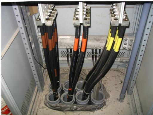
Another application where 400 amp sensors may be needed is with larger cable diameters such as aluminum conductors. If you are unsure, forward the sensor opening dimensions to the installer so they may choose the proper size.
