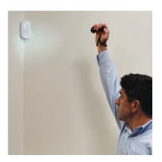
**Snap-Set Walk Test:** Triggers walk test mode with the flick of a flashlight, reducing the number of trips to the sensor during installation.
