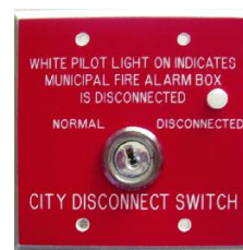
City Disconnect Switch
