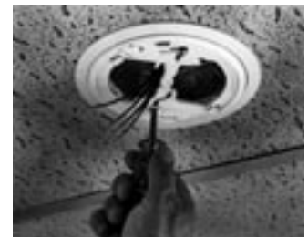
Figure 2. Install detector.
