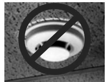
Figure 4. Detector without adapter bracket
