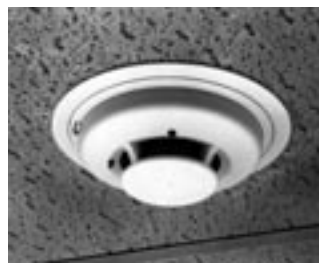
Figure 3. Adapter bracket covers previous detector footprints and flawed installations.
