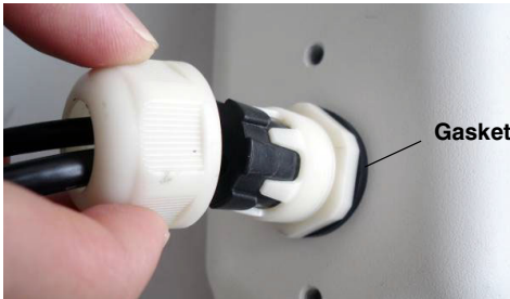
Figure 7 Ensure Conduit Plug Nut Is Tight
