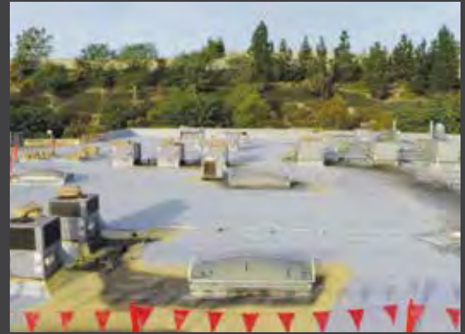
View of partially completed ccSPF installation
