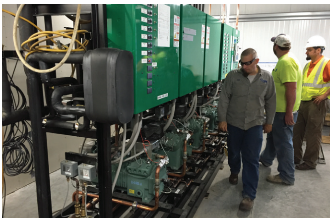
The team from Zero Zone, SCR and Coborn's make final adjustments to the low-temperature rack system.
