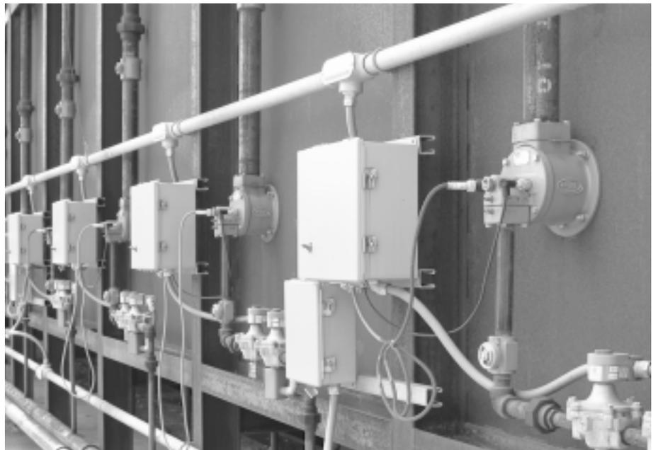
*Effective post-weld heat treating for stress relief plays a crucial role in the quality and reliability of SRS Wintergreen's processing equipment. For the new car-bottom furnace, the company selected Eclipse ThermJet burners to provide efficient, uniform and environmentally superior process heating.*
