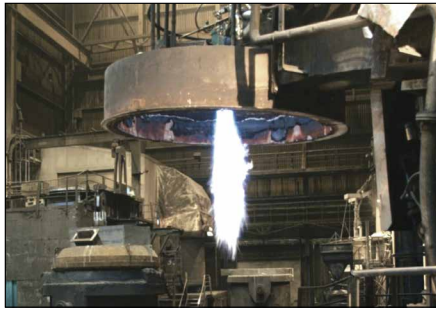
Vertical gantry type ladle preheating.
