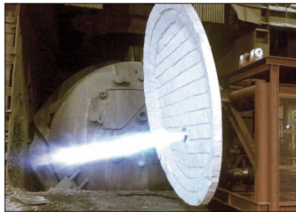
Horizontal type ladle preheating.
