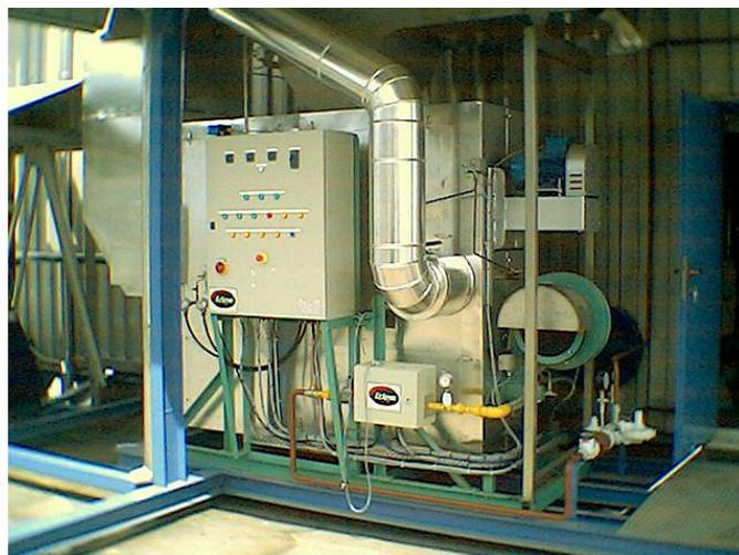
*Recirculating Indirect Fired Air Heater*
