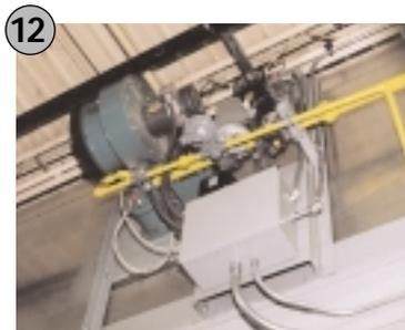
**Photo 11** Control panel for RatioMatic burner(s). Motor starters and other heat generating devices are kept in a separate cabinet.
