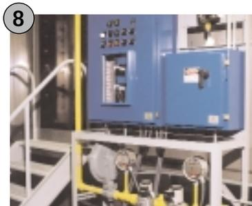
**Photo 7** 64IR burners in final stage of washer. Burners are configured in 4 zones providing 1.32 million Btu/hr.
