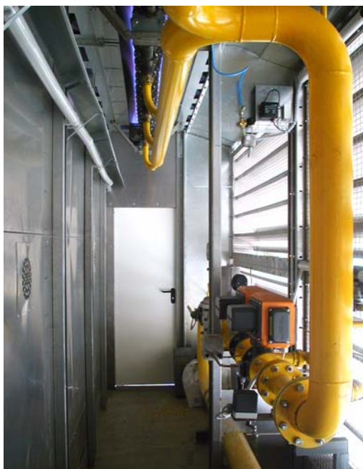
Direct air heating with NP- III AIRFLO® burners in continuous flow dryers for grain.
