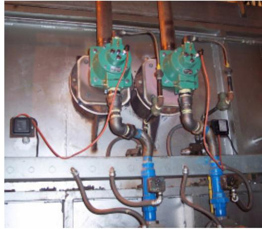
*Additional views of Eclipse AutoRecupe SER burners showing valving for pulse firing.*
