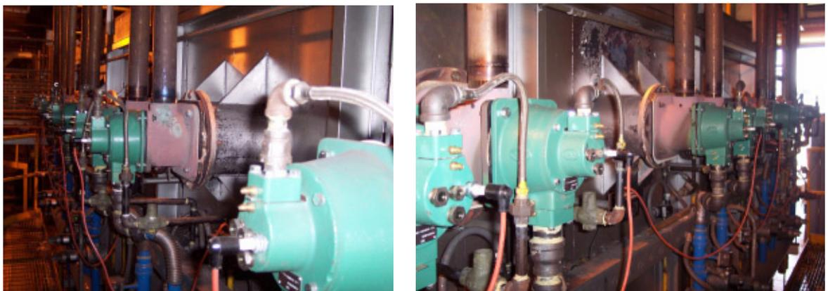
*Close-up views of Eclipse AutoRecupe SER burners installed on multi-purpose metal treating furnace.*
