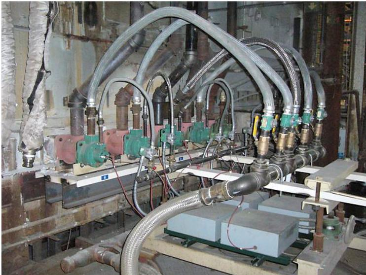
*Overall view of edge heating system installed on tin bath.*
