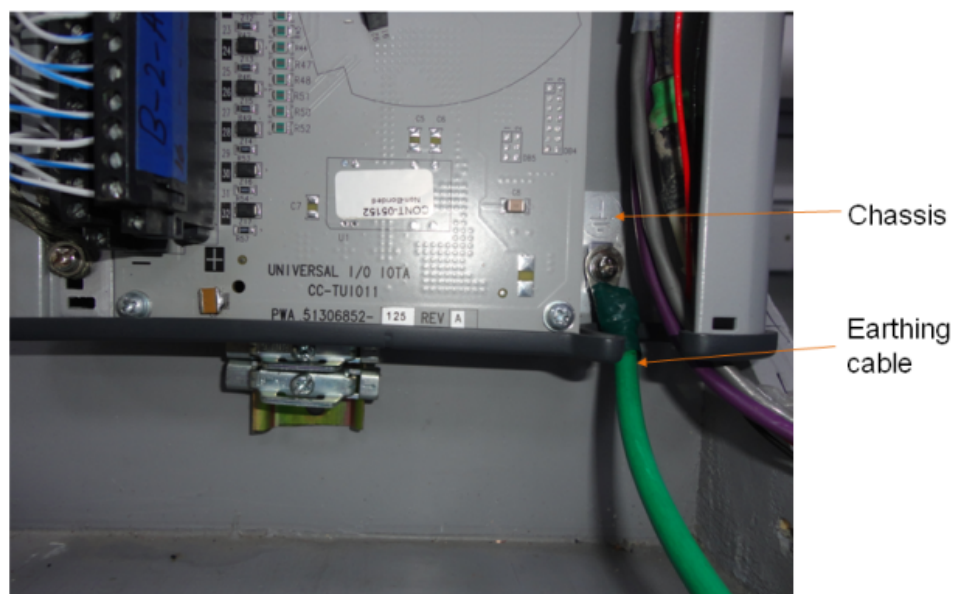
Figure 8.7 Grounding connections
