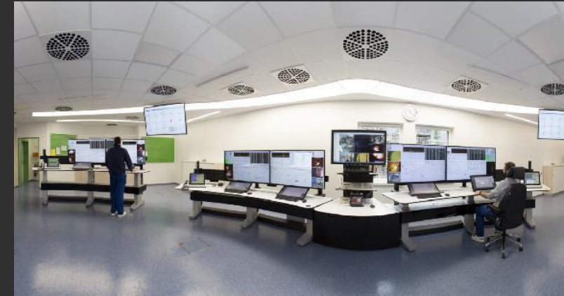
Control Room Operations Now
