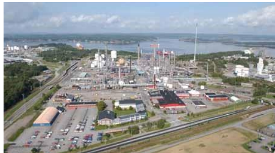
The Stenungsund cracker plant is one of the most flexible in Europe, using naphtha, ethane, propane and butane as feedstock.
