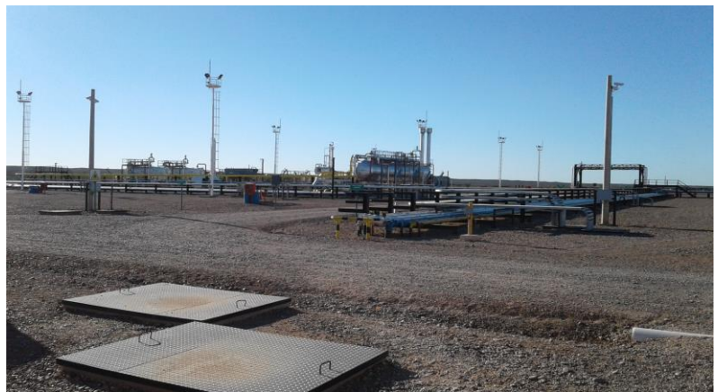
Shell's Early Production Facility in Sierras Blancas
