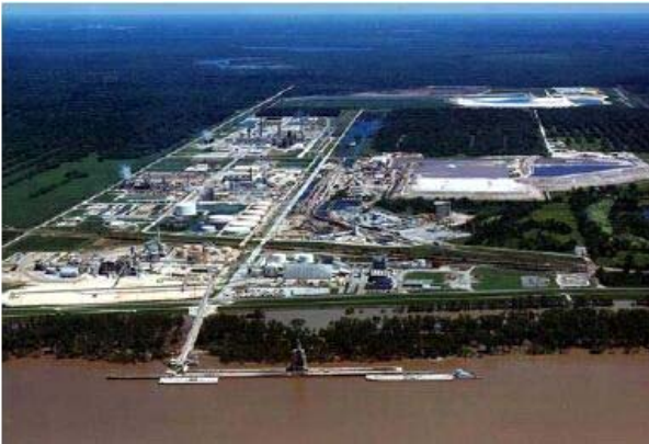
Honeywell chemical plant in Geismar, Louisiana
