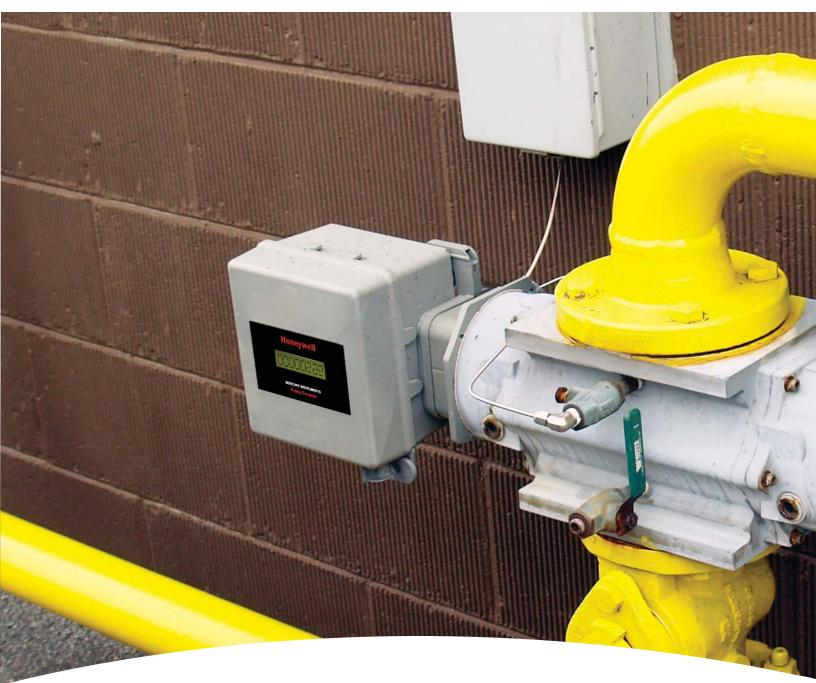
INTEGRAL, MULTI-METER ADAPTER PLATES ELECTRONIC BACKUP INDEX (REI) FOR UNCVOL
