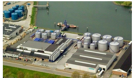
Transnational Site and Storage Tanks
