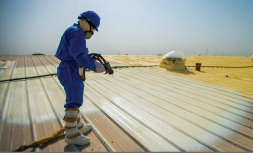
Spray foam was applied over the metal roof to prevent leakage and increase energy efficiency.
