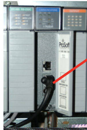
Figure A-4. DF1 Connection to RJ45 Socket
