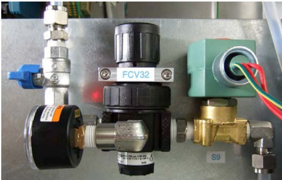
Figure 21. Venturi Supply (Option)
