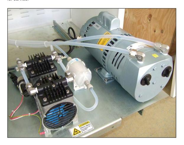
Figure 12. Mechanical Pump Assembly
