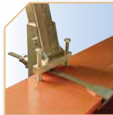
Stanchion installation complete
