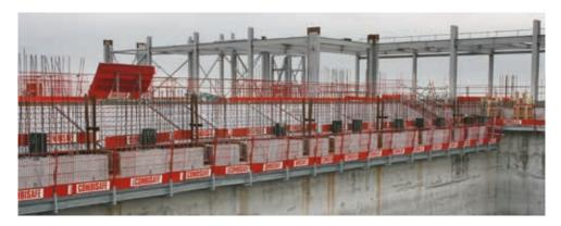
This light weight system comprises a console, which is suspended or attached to the structure using a range of supports, into which a boardwalk is fixed to create a walkway. The consoles also support Safety Posts and Barriers from the edge protection system on the outside of the walkway.
