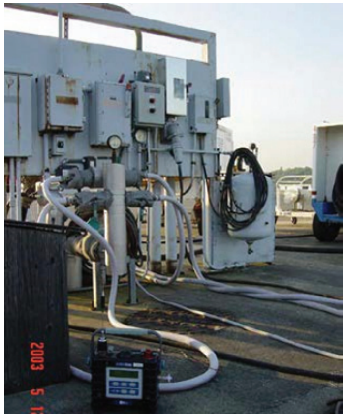
Figure 4. AreaRAE monitoring mechanical equipment.
