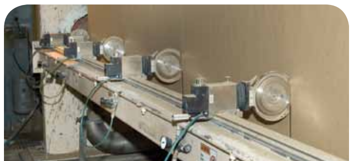
Figure 5. Cutting and slitting
